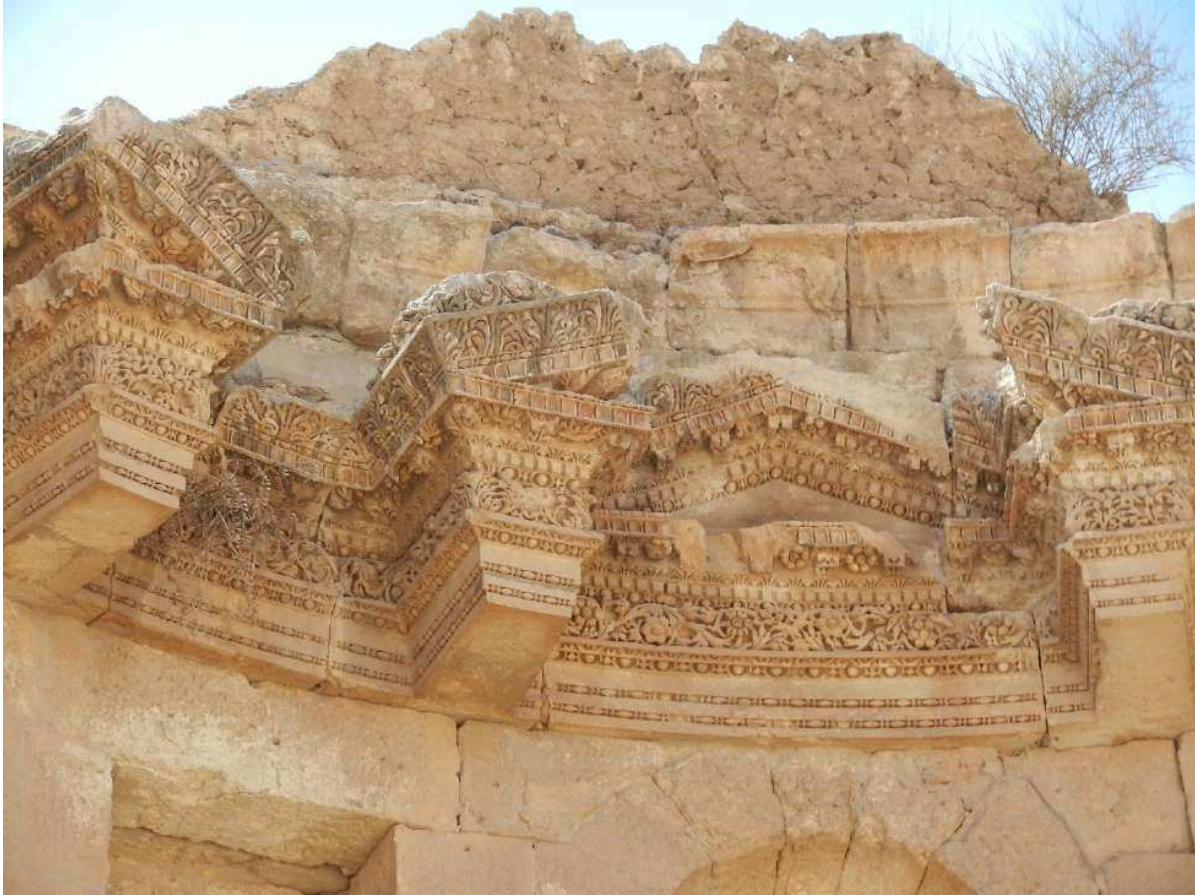
Figure 6.6- Closeup of Jerash Nymphaeum showing intricate detail of the façade. Photograph by T.R. Paradise (2007).
