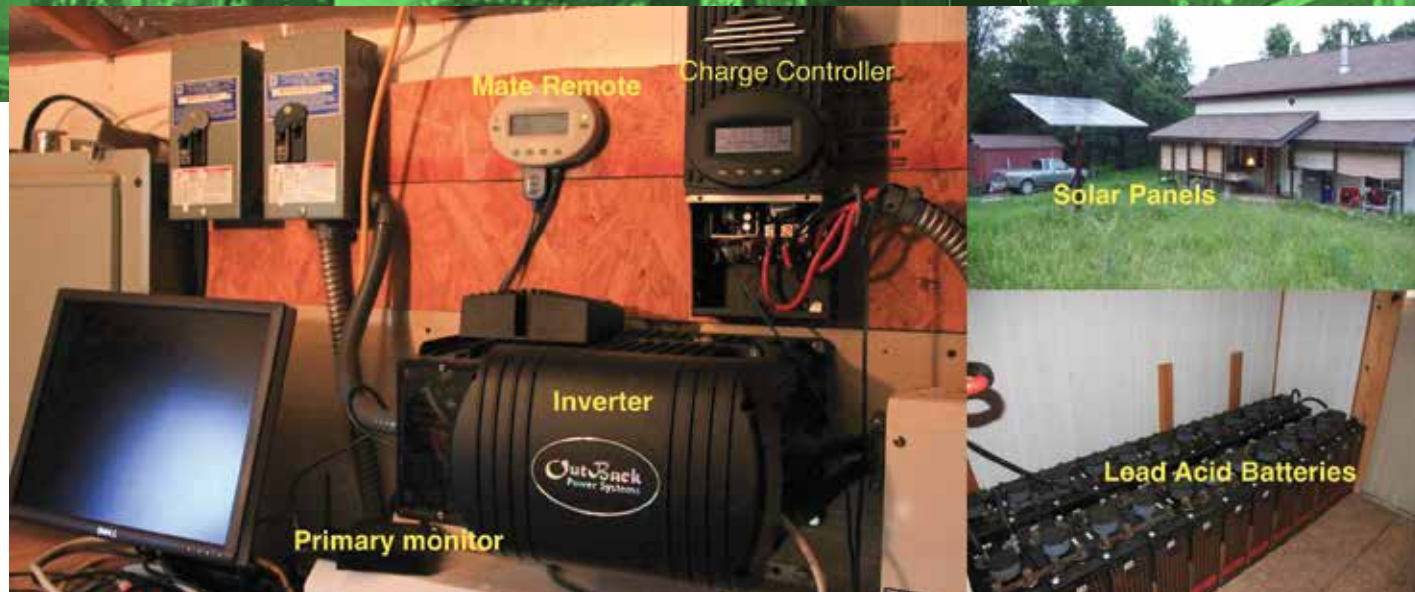
This prototype measurement system in an off-grid home in Arkansas helps the researchers understand how energy is generated and consumed in homes powered by renewable sources.
