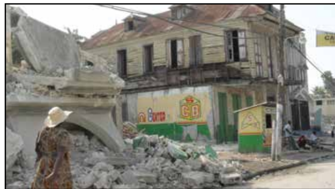
Above: In a heavily damaged area of Port-au-Prince, Cox found standing wood-framed structures next to reinforced concrete structures that collapsed.
