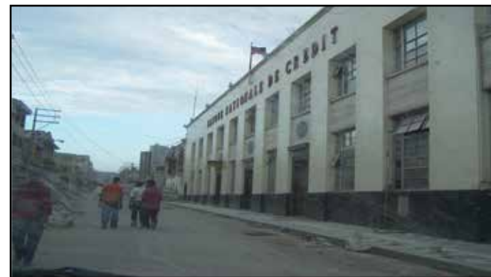
Above and right: In the same area of intense damage and destruction, some structures, probably built with features included in the International Building Code, suffered little or no damage.
