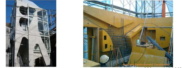
Figure 4: Akutawaga Westside Project
