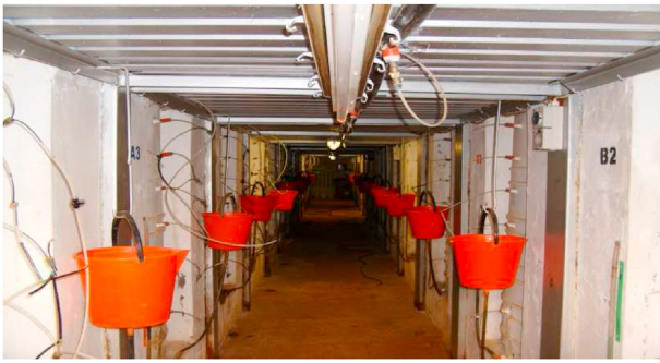
Figure 2. Underground chamber of the lysimeter unit showing that each lysimeter has a manometer through which the height of the water table is regulated by recharging from a bucket.
