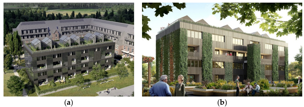
Figure 3. NBS implementation of Green Wall and Green Roof within CLEVER-cities case study 'Fischbeker Höfe' in Hamburg/Germany: (a) southview, (b) northview © DeepGreen Development.
