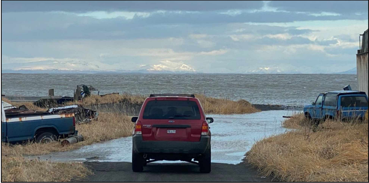
Figure 40. A flooded road near the retaining wall on the east side of the community. This stretch of coastline floods regularly during high storm-tides. Image provided by Angela Johnson, November 2020.
