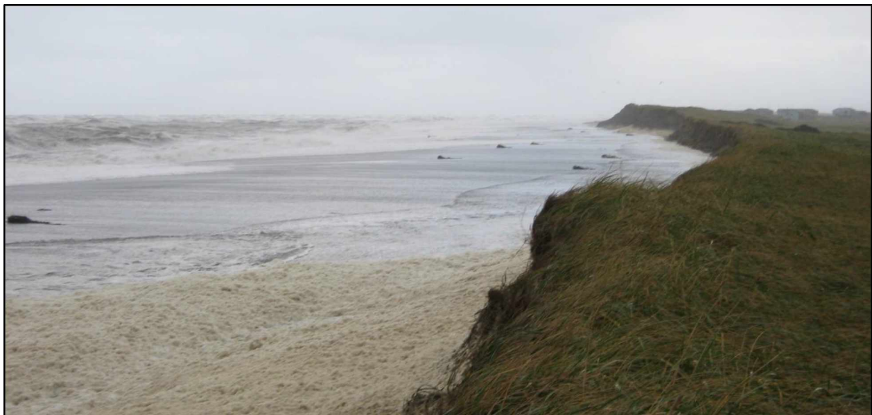
Figure 42. Photograph taken from the solid waste disposal site looking towards the community on the ocean side of the spit. As the bluff face erodes, sediment at or near the vegetation line is removed and there is an increase in the slope of the dune toe as it retreats landward. October 2018.
