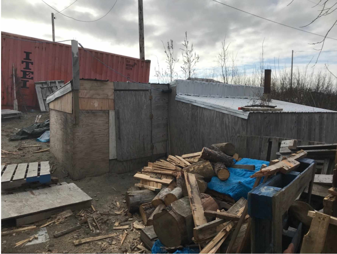
Figure 17: A maqivik . The door on the left leads to the cooler side for undressing and relaxing, and section with the lower roof and chimney is the hot area with the stove. The abundance of wood indicates it is well used. The red shipping container behind it is the shop. Bethel, April 2019. Photo by Ellen Carrlee.
