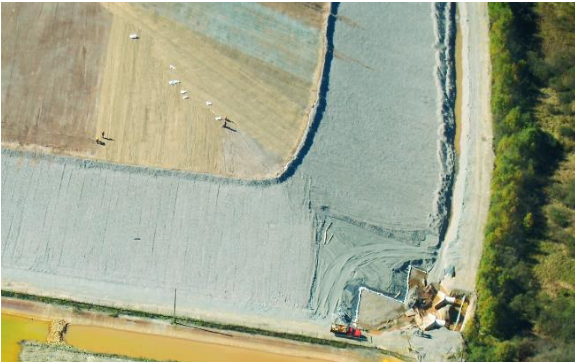
Figure 1-1: Engineered cover system being installed over a waste rock pile (WRP).
