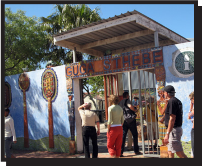
Langa Township, Cape Town, Guga S'Thebe, a combined tourist and community centre
