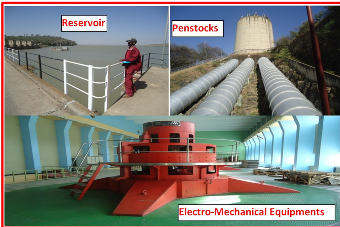
Figure 3.8 Few features of Koka Hydropower Plant
