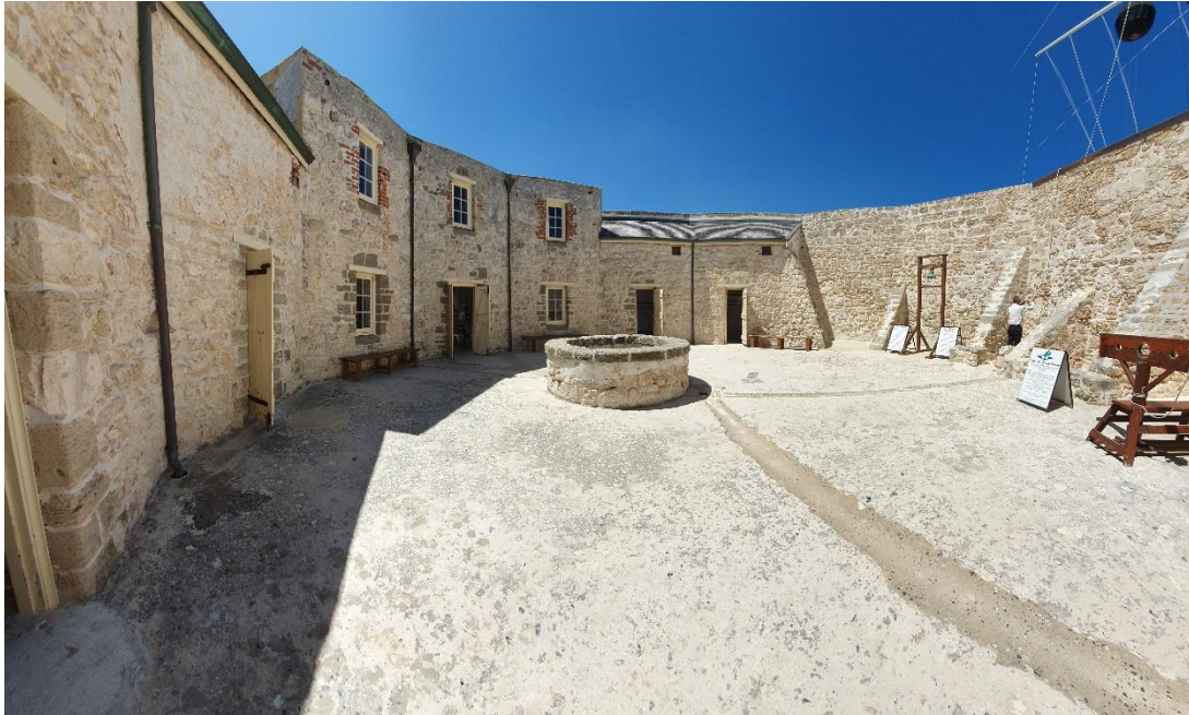
inspection principle was central to Bentham's prison, the gaol may be considered a colonial adaptation of the model. 33 Figure 3 The interior of Fremantle Gaol showing the gaoler's quarters (centre) and surviving cells (left and right) 34
