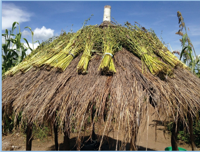
Grass being used in roof construction, Bidibidi.
