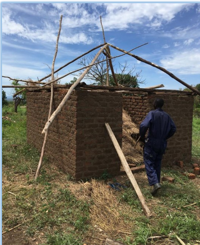
House constructed of unburnt bricks, Bidibidi.
