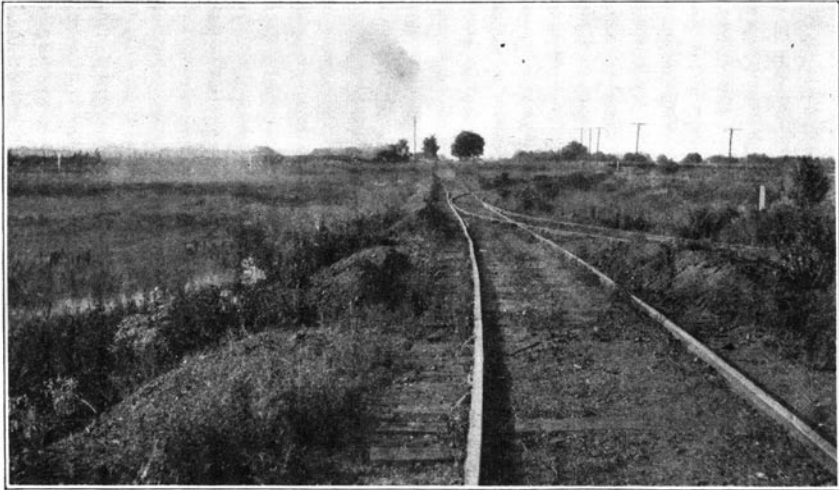
FIG. 16. DISTURBANCE OF GRADE BY SUBSIDENCE.
