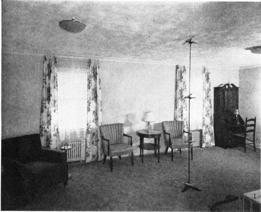
FIG. 2. VIEW OF LIVING ROOM IN I=B=R RESEARCH HOME
