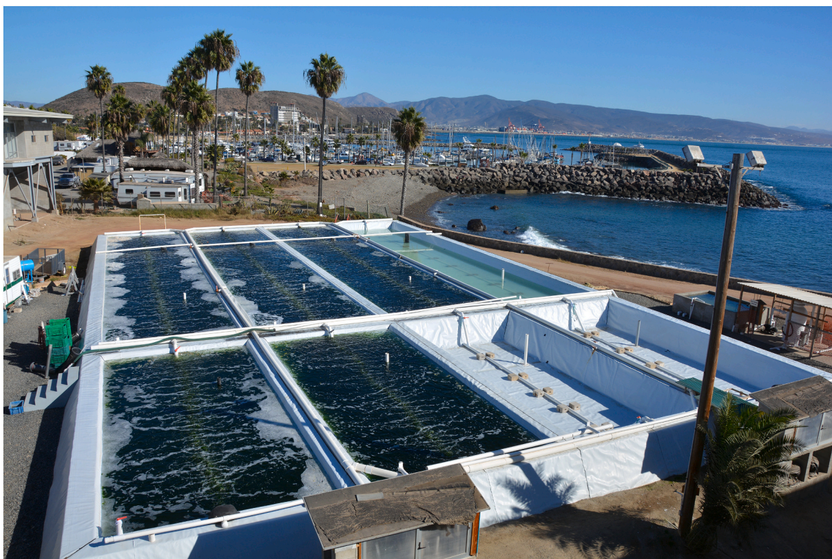
Fig. 1. Land-based ponds for U. ohnoi cultivation at the Autonomous University of Baja California (Ensenada, Baja California, Mexico). Cultivation method consists of “tumble culture” with aeration from the bottom of the pond. Uniquely the four smaller ponds of 40 m 3 were used for the study.
