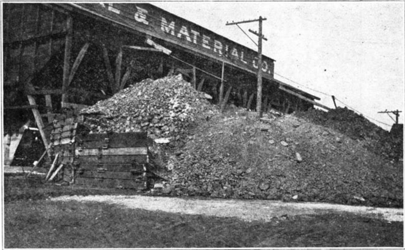
FIG. 25. VIEW OF COAL PILE SHOWING TIMBER RETAINING WALL ANCHORED INTO COAL PILE BY WOODEN SUPPORTS
