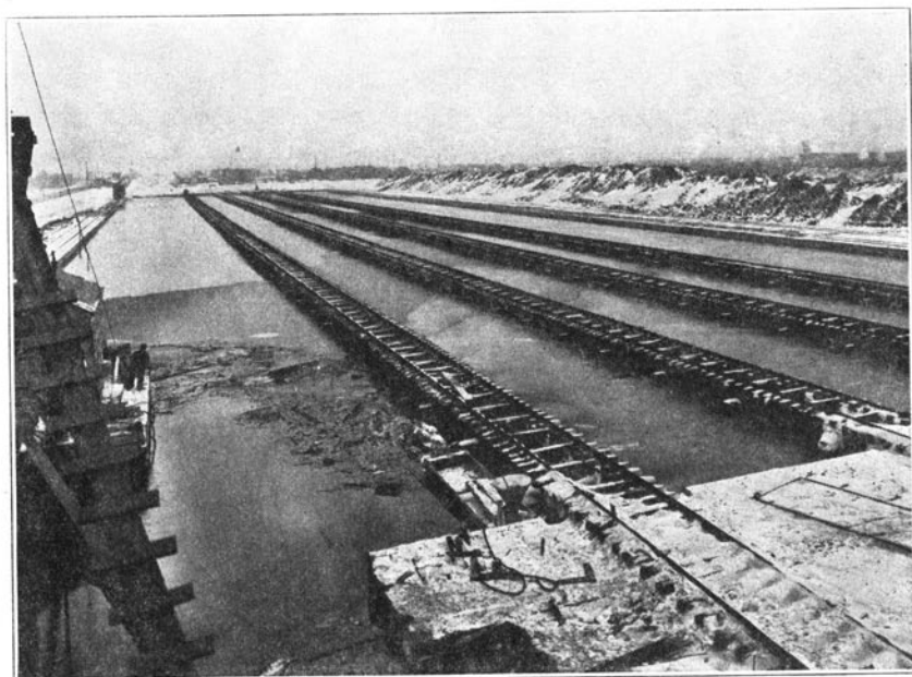
FIG. 72. UNDERWATER COAL STORAGE PLANT OF THE STANDARD OIL COMPANY, WHITING, INDIANA (100 000 TONS CAPACITY)
