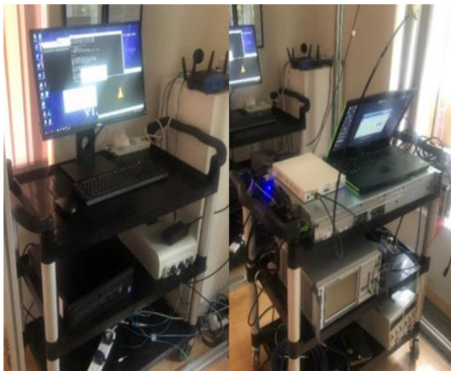
(a) Intelligent Home IP Gateway, Layer 2 Processor & DRAN
