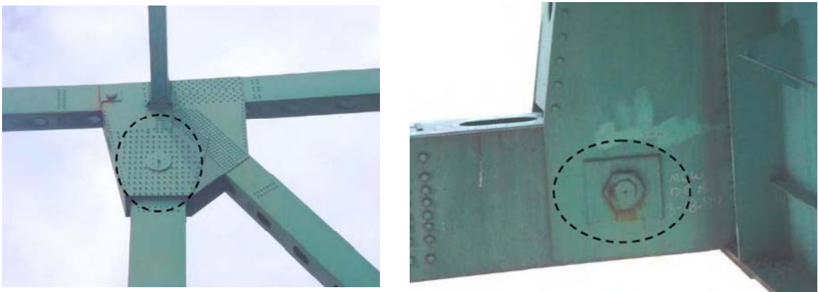
Figure 4.43 Truss intermediate hinges
