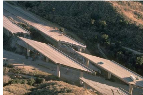
(b) Gavin Canyon Undercrossing
