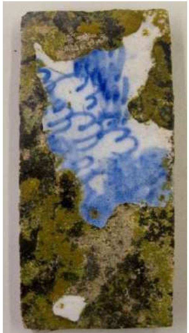
Biological degradation on tile H3
