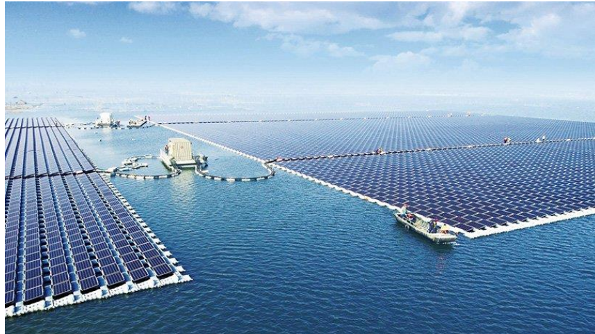
Figura 13 – Sungrow Huainan Solar Farm (Designboom, 2018).
