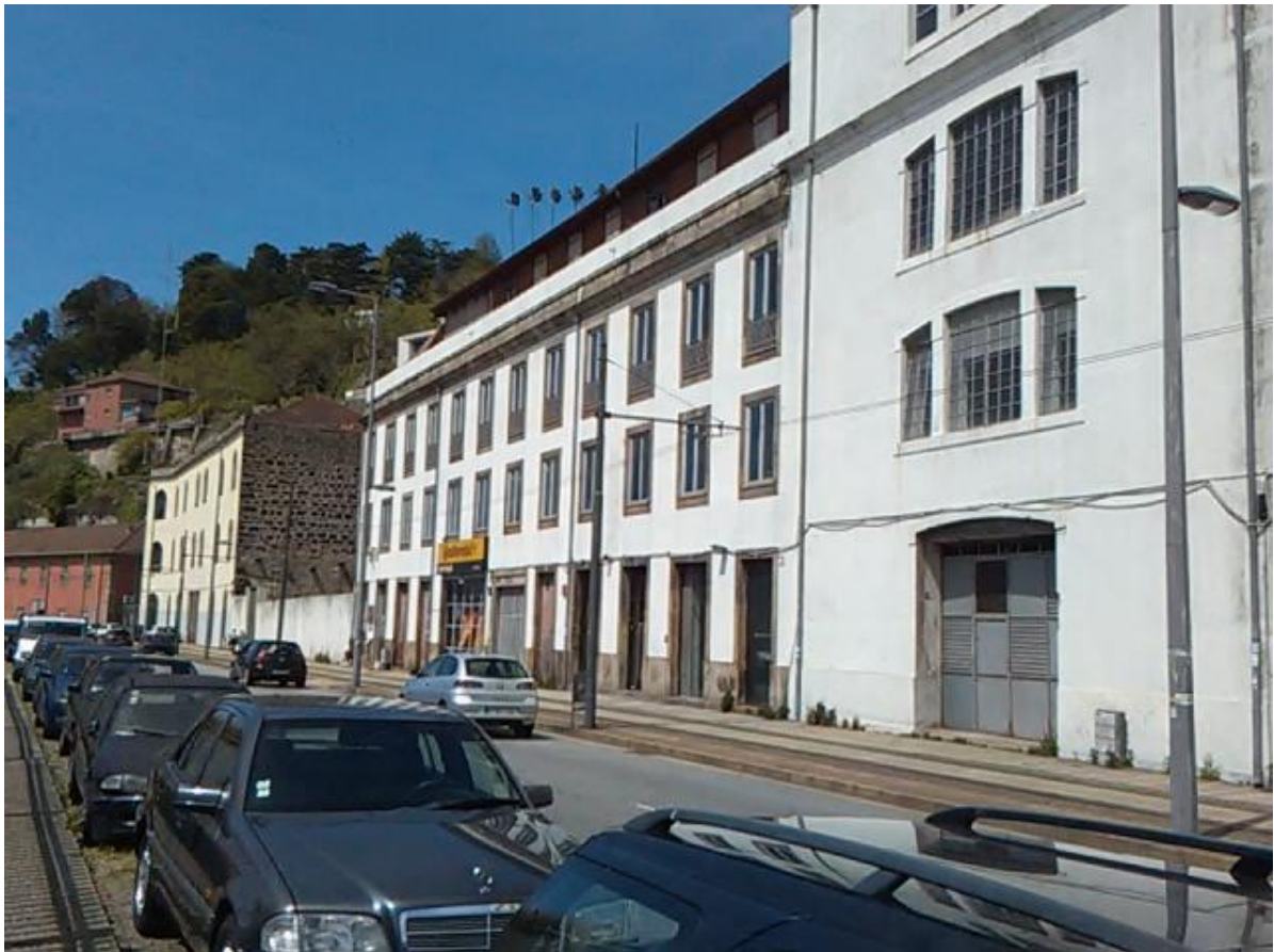
Figure 5.3 General view of the building where the Lottus is situated on Rua de Monchique by the Douro river (photograph of the author, 2016).
