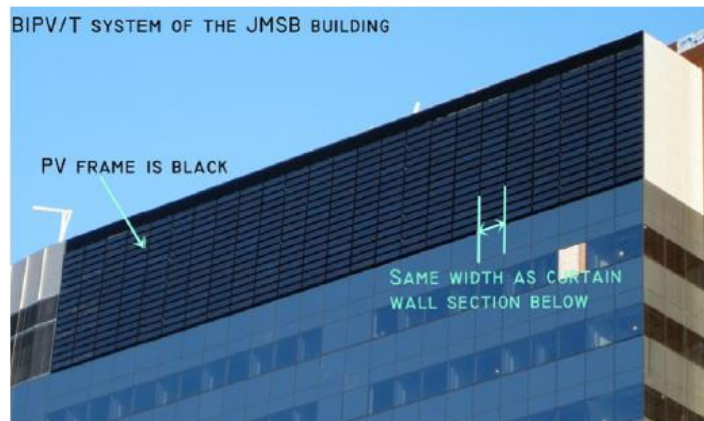
Figure 12: BIPV/T System of the JMSB Building [24]
