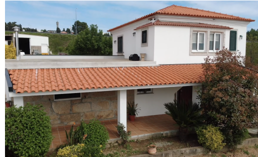
(b) Building Front View
