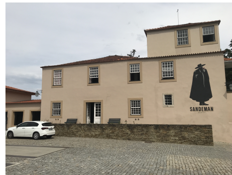
(b) Building Front View
