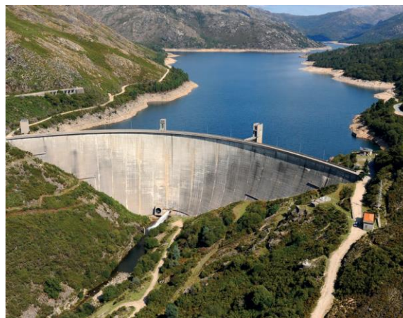
Figure 25 – Vilarinho das Furnas dam (EDP 2016).
