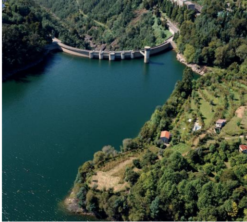
Figure 24 – Caniçada dam (CNPGB 2016).
