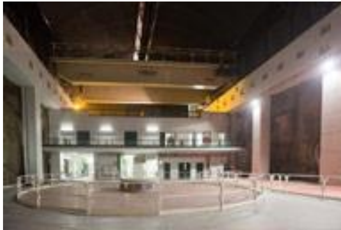
Figure 23 – Salomonde II power station (CNPGB 2016).
