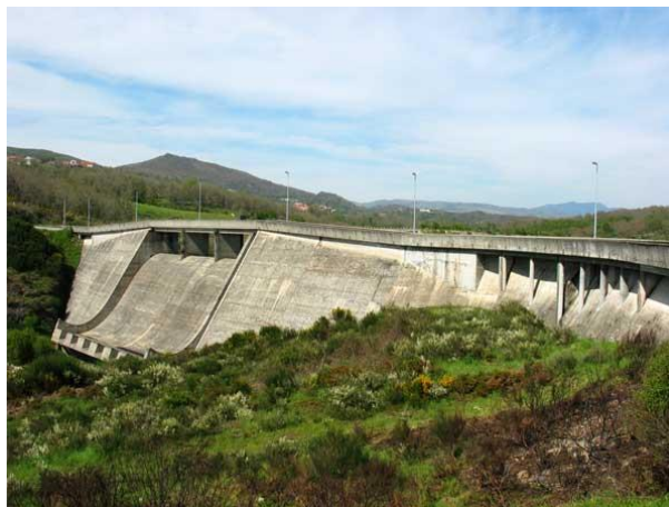
Figure 16 – Alto Cávado dam (CNPGB 2016).
