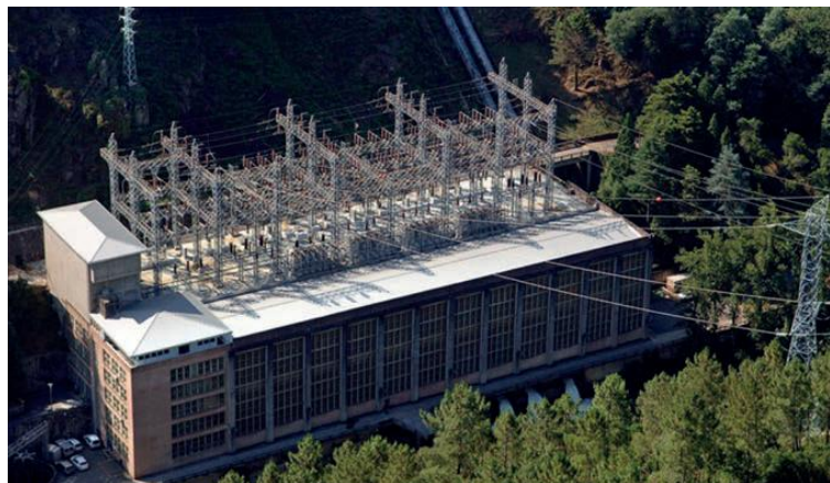
Figure 18 – Vila Nova power station (EDP 2016).
