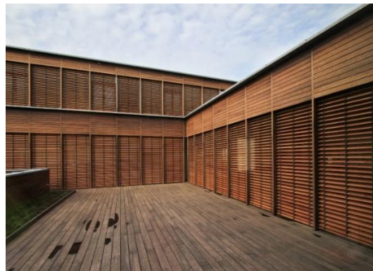
Figure 4.14 - Example of Exterior Blinds [79]
