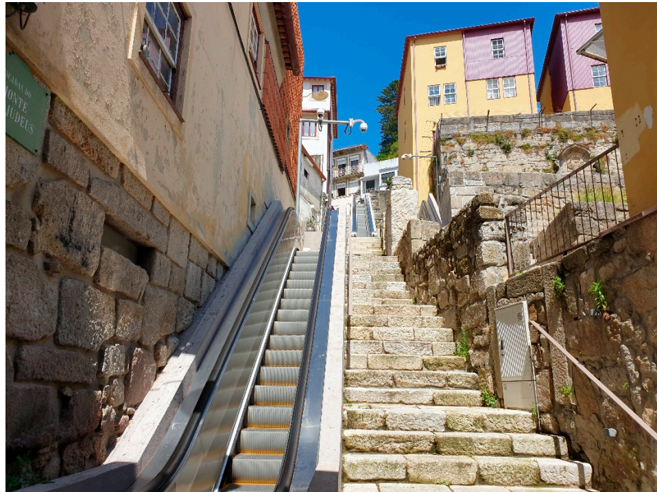
Figure 5. Recently installed escalators at Porto's historic centre.
