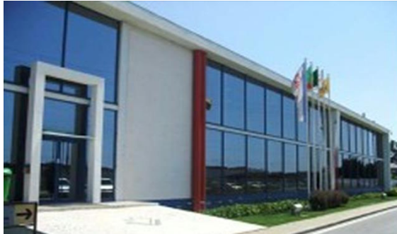
Figure 1.2 – Entrance building of Bosch Thermotechnology S.A. in Aveiro.
