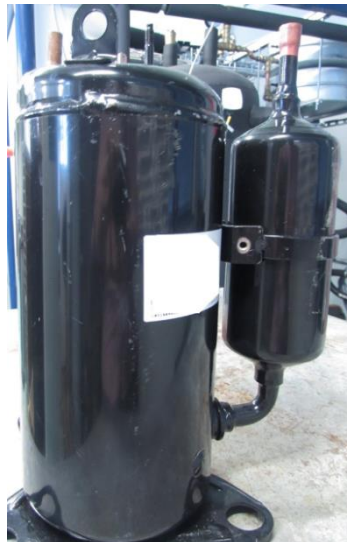
Figure 5.8 – Fixed speed rotary compressor.
