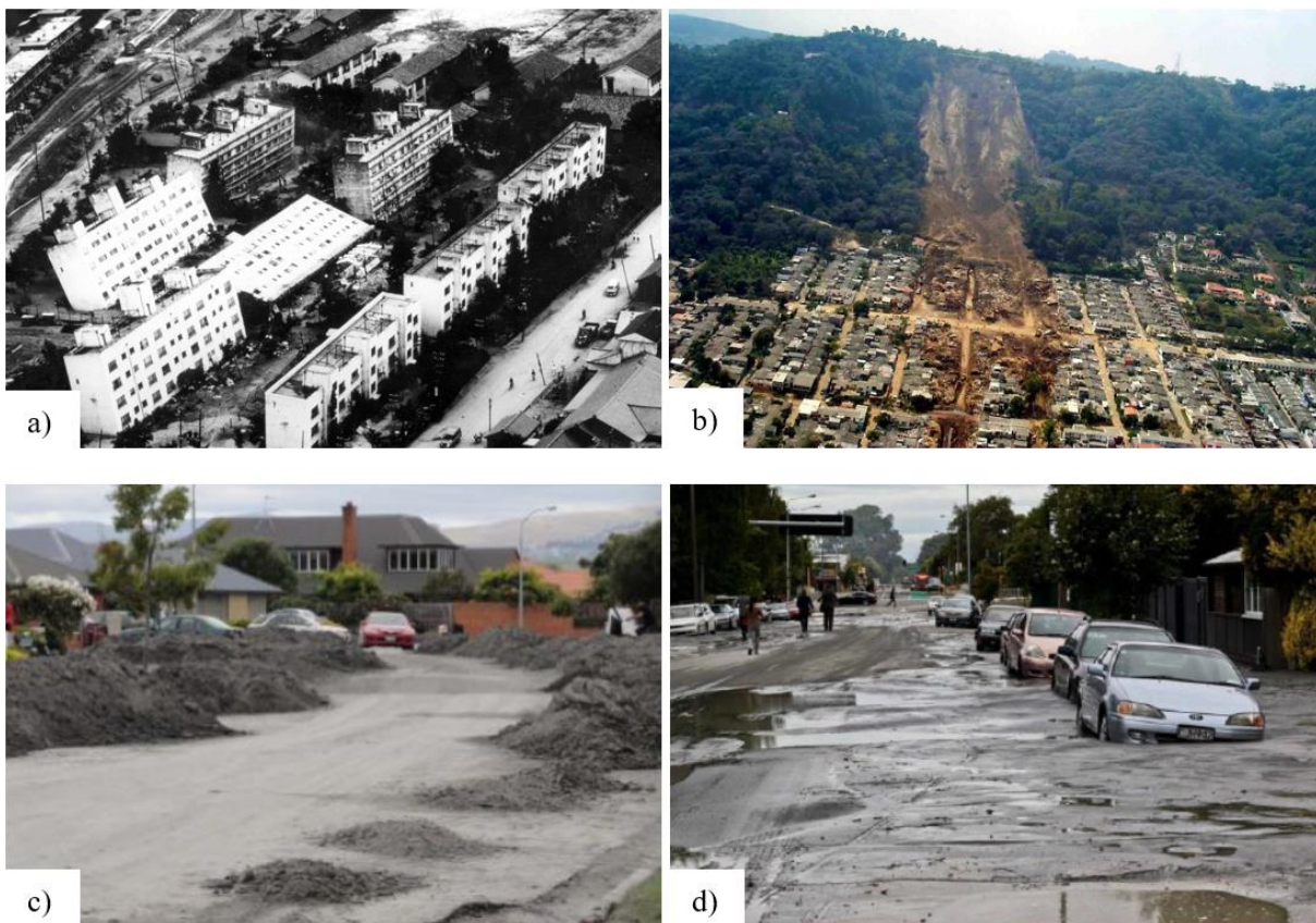
Figure 2.1 – Liquefaction-induced damage: a) Tilted buildings during Niigata Earthquake in 1964 (USGS, 2020a); b) Landslide caused by El Salvador earthquake in 2001 (USGS, 2020b); c) and d) liquefaction in residential areas (Cubrinovski et al., 2011)
