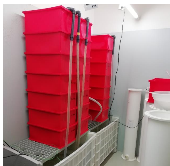
Figure 14 - Tricking filters - biofilter activation systems in BOGA.
