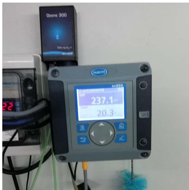
Figure 19 - Ozone generator and the display monitor of the redox potential and temperature probe.
