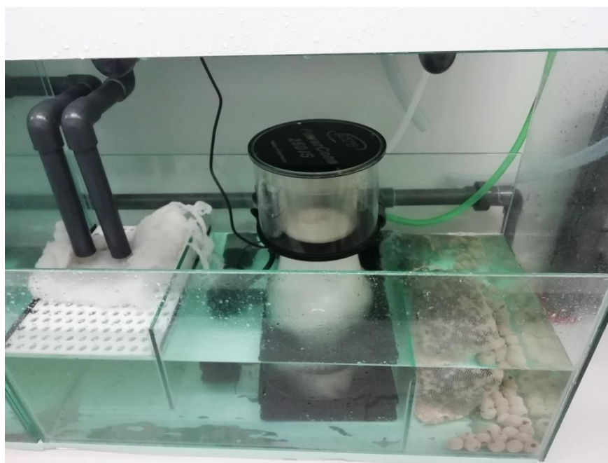
Figure 37 - Sump components in challenge room p.14: mechanical filter (left), protein skimmer (centre), biofilters (right).
