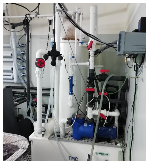
Figure 31 - TMC filtration system in aquaculture room p.20.
