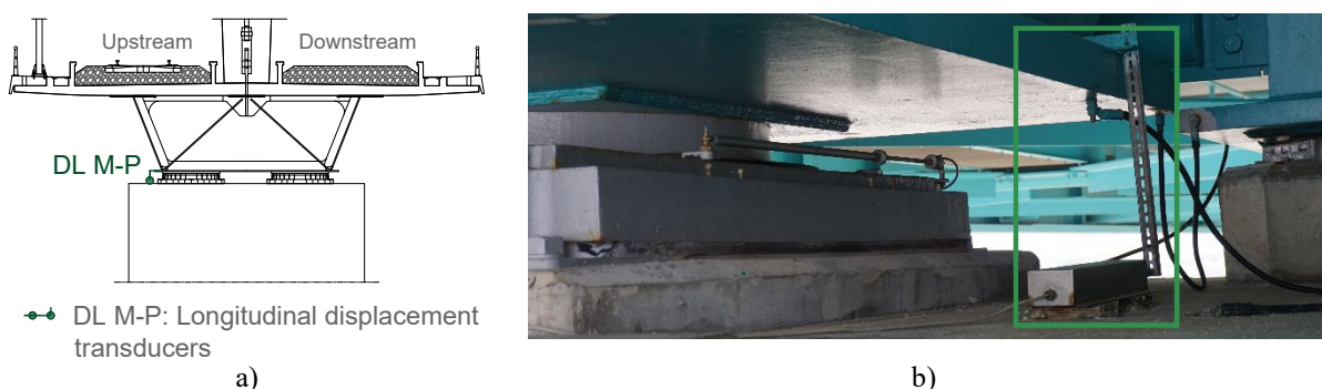
Figure 3.17 - Longitudinal displacement transducer (DL): a) cross section location, b) sensor installation.
