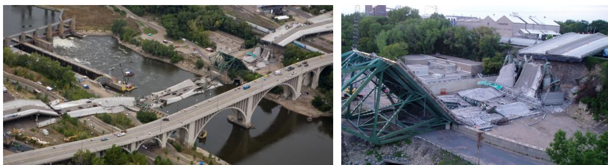
Figure 2.4 - Collapsed north section of the Minneapolis I-35W Bridge, USA, in 2007 (WordPress, 2016).
