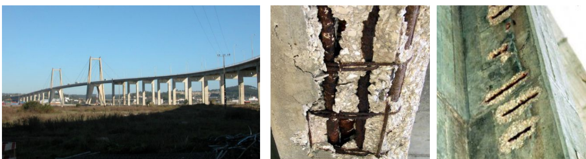
Figure 2.7 - Corrosion of the reinforcement bars in Edgar Cardoso bridge (Armando Rito Engenharia, 2016).
