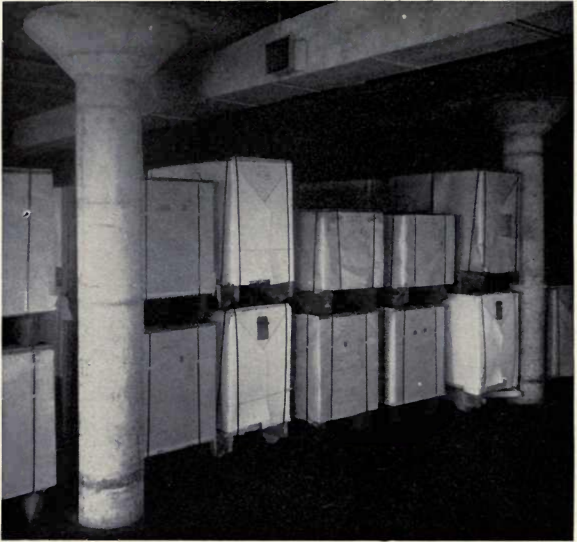
Fig. 7.—At the carton factory, paper for milk containers is stored in large rooms. Before the air enters the room it is washed, humidified, and heated to a uniform temperature. Note ventilator.
