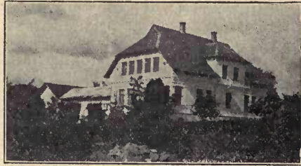
TOWN DAIRYMAN'S HOUSE AND COW STABLE.
