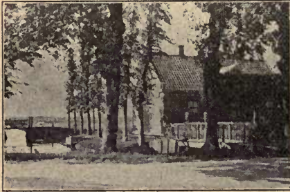
SHOWING THE USUAL LOCATION OF A HOLLAND HOME. THE BRIDGE, AFFORDING A COMMUNICATION BETWEEN THE ROAD AND HOUSE, IS CLOSED IN THE MIDDLE WITH A GATE.
