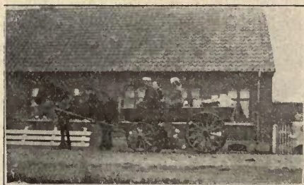
RETURNING FROM MILKING COWS AT TETHER. LABORER'S COTTAGE IN BACKGROUND.
