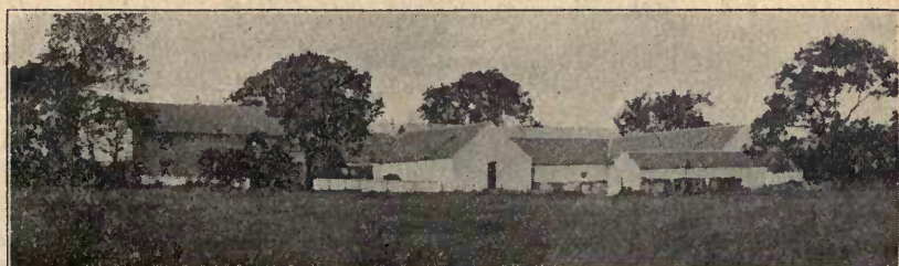
BUILDINGS ON AN AYRSHIRE DAIRY FARM. IN THIS CASE THE STABLING FORMS THE SQUARE COURT AND THE HOUSE IS OUTSIDE, BUT ADJACENT.
