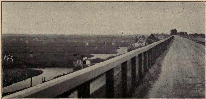
ROAD ON TOP OF THE DYKE RUNNING AROUND THE ZUIDER ZEE. THE WATER IN THE SEA ON THE RIGHT IS 12 TO 15 FEET HIGHER THAN THE LAND ON THE LEFT. NOTICE MEADOWS DOTTED WITH CATTLE.
