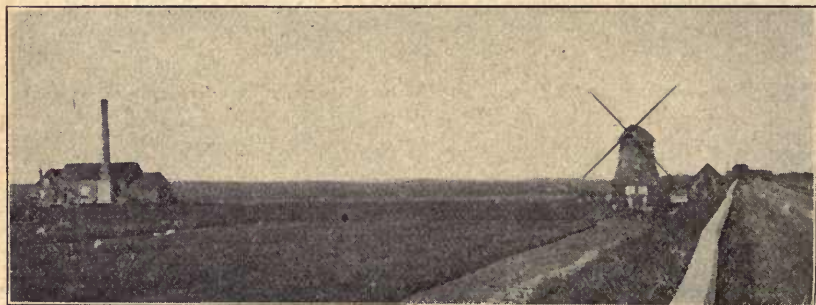
WINDMILL AND ENGINE HOUSE USED FOR PUMPING WATER FROM CANALS INTO THE ZUIDER ZEE ON RIGHT. A LARGE STORAGE RESERVOIR EXTENDS FROM THE MILL BEYOND THE ENGINE HOUSE. THIS CONTAINS A RESERVE WATER SUPPLY, AND IN DRY TIMES CAN BE LET BACK INTO THE CANALS IF DESIRED FOR IRRIGATION PURPOSES. SEA WATER CANNOT BE USED ON ACCOUNT OF THE SALT.
