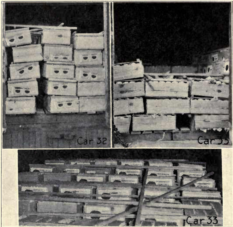
FIG. 10.—IMPROPERLY BRACED TOMATO LOADS
