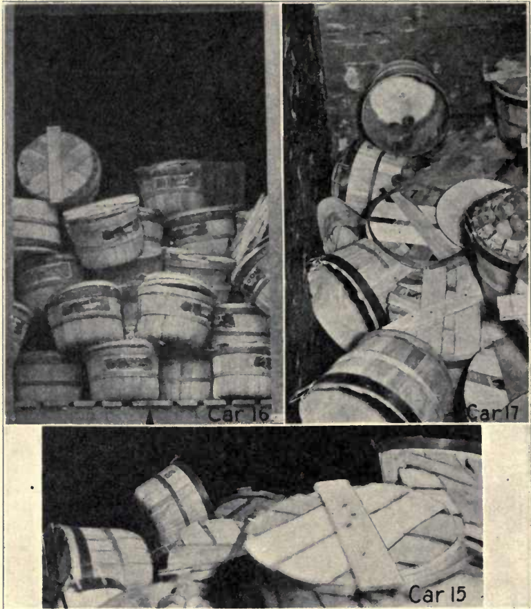
FIG. 5.—THE RESULTS OF LOOSE LOADING OF HALF-BUSHEL CONTAINERS OF PEACHES
