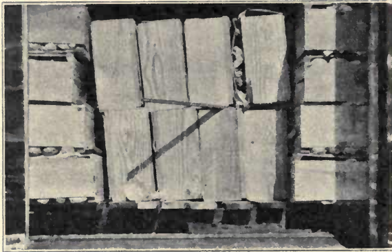
FIG. 12.—FAULTY LOADING AT DOORWAY
