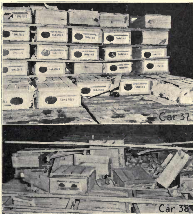
FIG. 13.—FURTHER EXAMPLES OF IMPROPER CENTER BRACING
