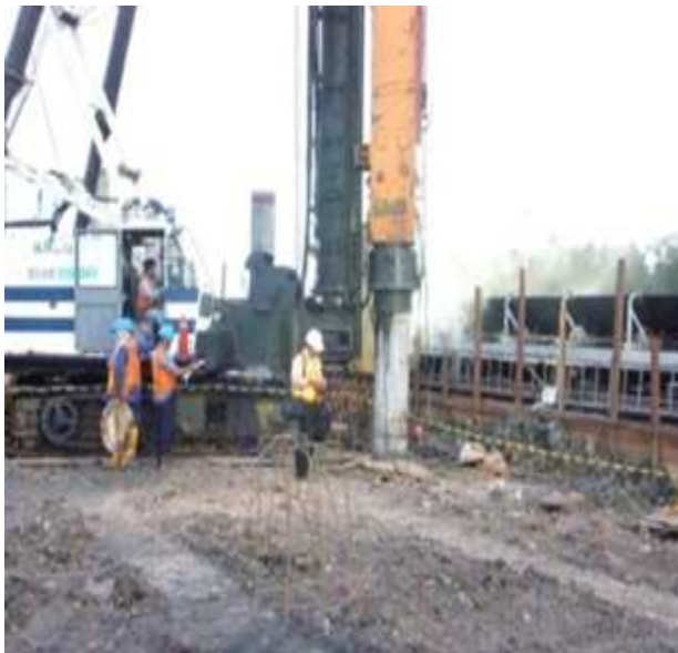
Figure 6. Pile driving in conveyor area
