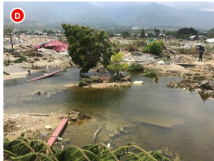
(b) Some water inundation appeared after the event, showing that the groundwater level in this area is high (Balaroa).
