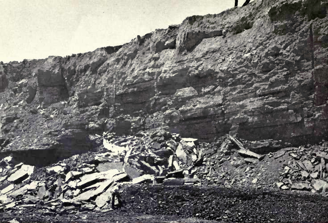
Overburden of No. 6 coal in Saline county often carries a high proportion of massive stone, mainly sandstone and limestone. (Fig. 9)
