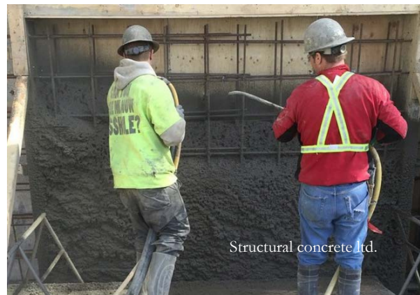
Figure 1.6: Pre-construction panel sprayed using the wet-mix process and an air lance
