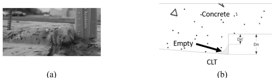
Fig. 10. (a) Photo of the rounded shape of the concrete notch due to the plastic film; (b) Definition of the reduced depth D'_n of the notch.
