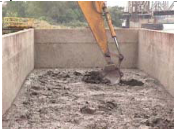
Fig. 6. A three cubic yard excavator removing sediment from the barge. The top layer has begun to dry and form a thin crust.
