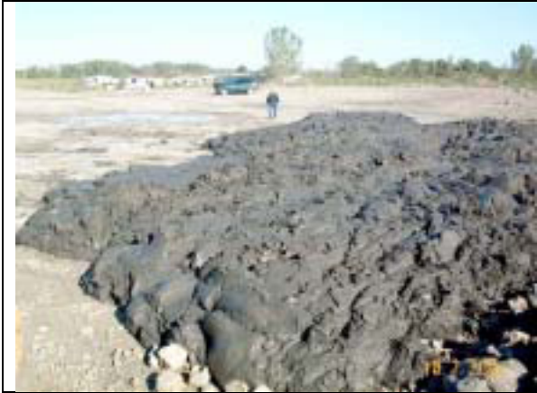
Fig. 21. Trucks were able unload sediment in contiguous piles demonstrating the ability to form a continuous layer about two feet thick.
