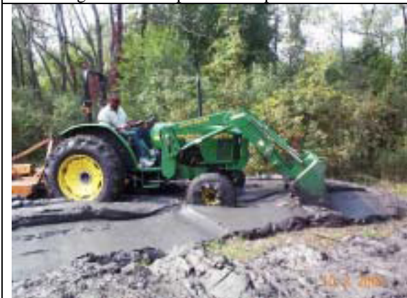
Fig. 13. The material was stiff enough to allow an endloader to spread it without using a form.
