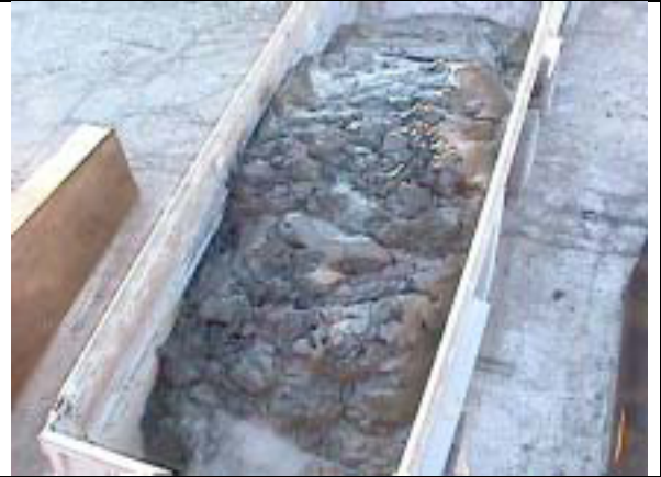
Fig. 10. The sediment maintained its consistency and piled inside the trucks.
