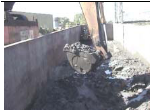
Fig. 7. The dredged material handled well in the bucket and maintained its consistency.
