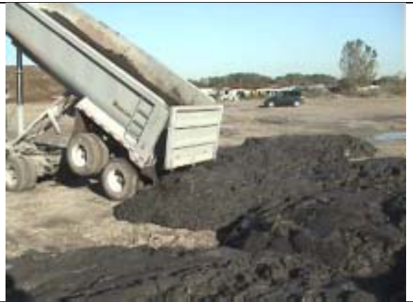
Fig. 16. Material being placed on the clay liner at the landfill.
