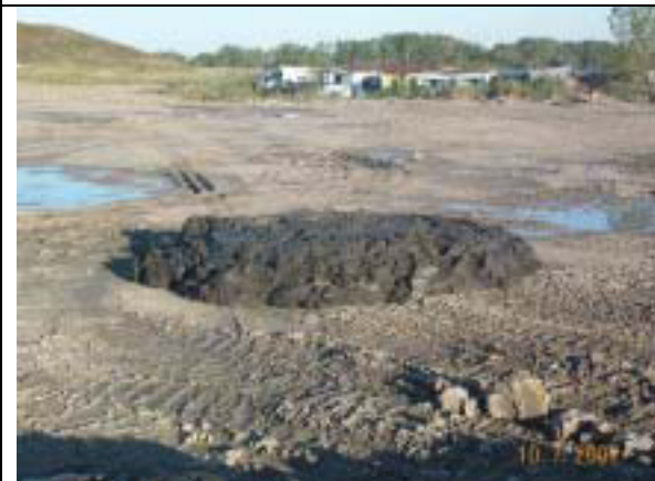
Fig. 19. As at the Powers site a week earlier, material formed piles at the landfill when dumped in one spot.
