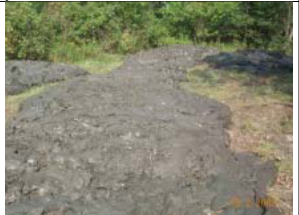
Fig. 12. A moving truck left a long pile with a height dependent upon the speed of the truck.
