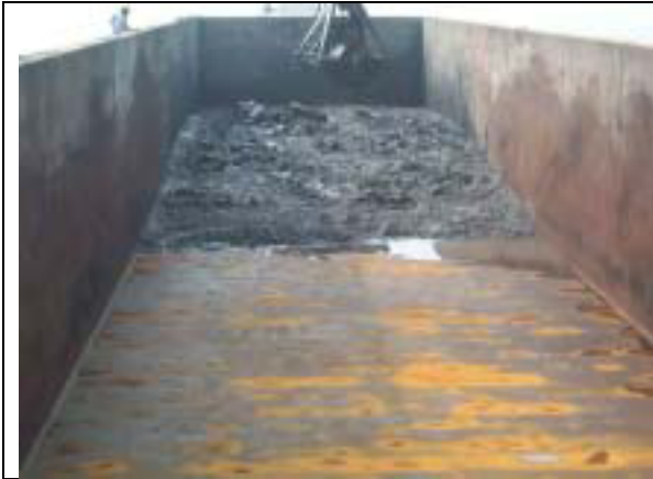
Fig. 3. Sediment is placed in a barge on Lower Peoria Lake on September 27, 2002. A clam shell bucket is used to minimize free water.
