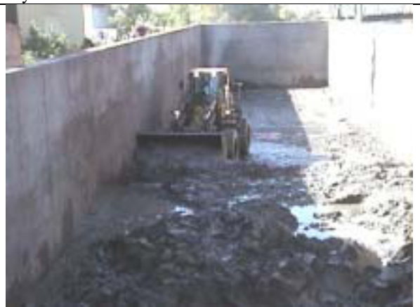
Fig. 8. Later in the day an endloader inside the barge pushed material into a pile to assist the excavator.
