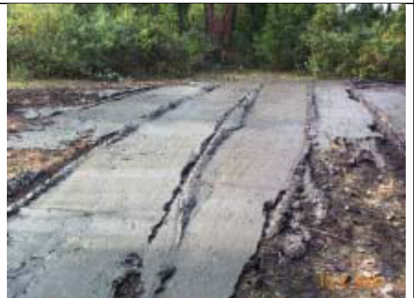
Fig. 14. Sediment spread to a depth of about six inches on the day it was deposited at the Powers site.
