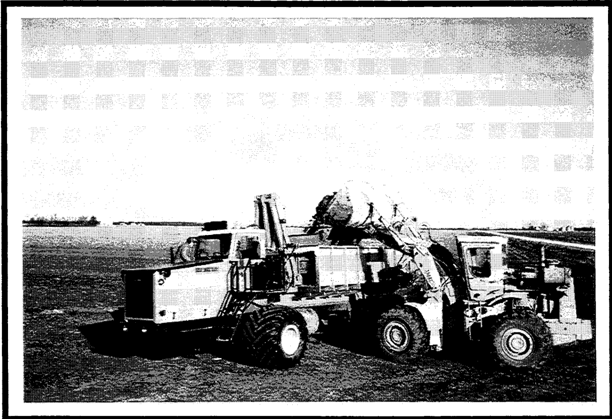
Figure D-1: An end loader fills the box of the modified sludge spreader prior to starting another round of soil spreading.
