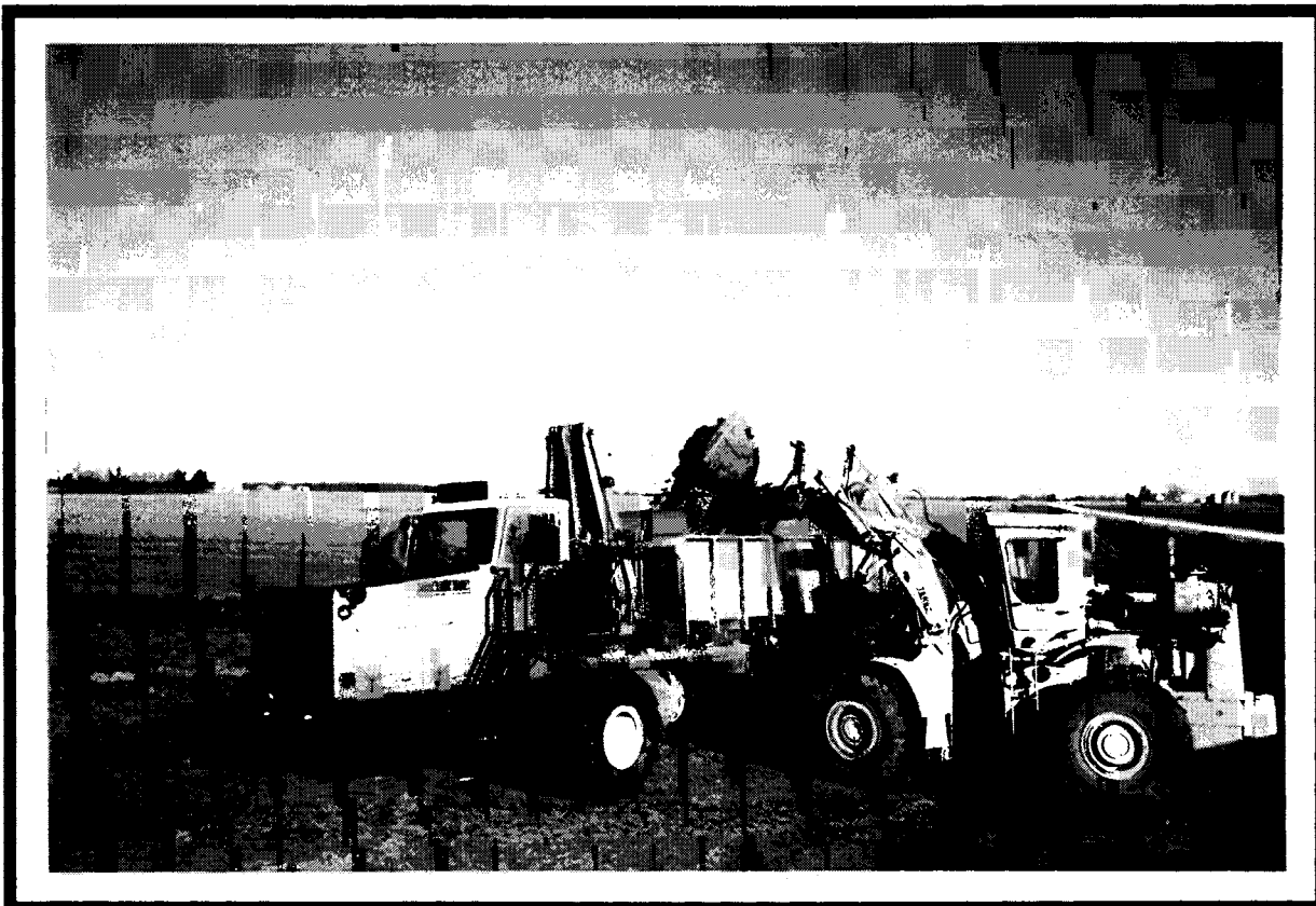
Figure D-1: An end loader fills the box of the modified sludge spreader prior to starting another round of soil spreading.
