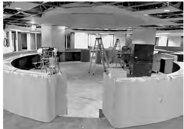
Newsroom under construction. (Photo by Washington Post)
