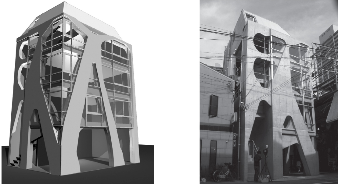
Figure 2.1: Akutagawa River Side office building (Ohmori et al., 2005)
