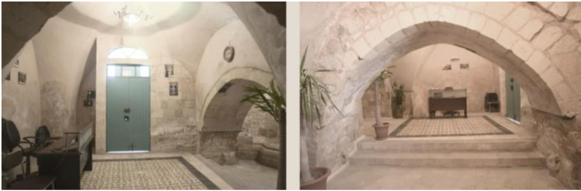
Figure 4.22 Examples of the vaulted roof system found in many of As-Salt vernacular dwellings (By Author)
