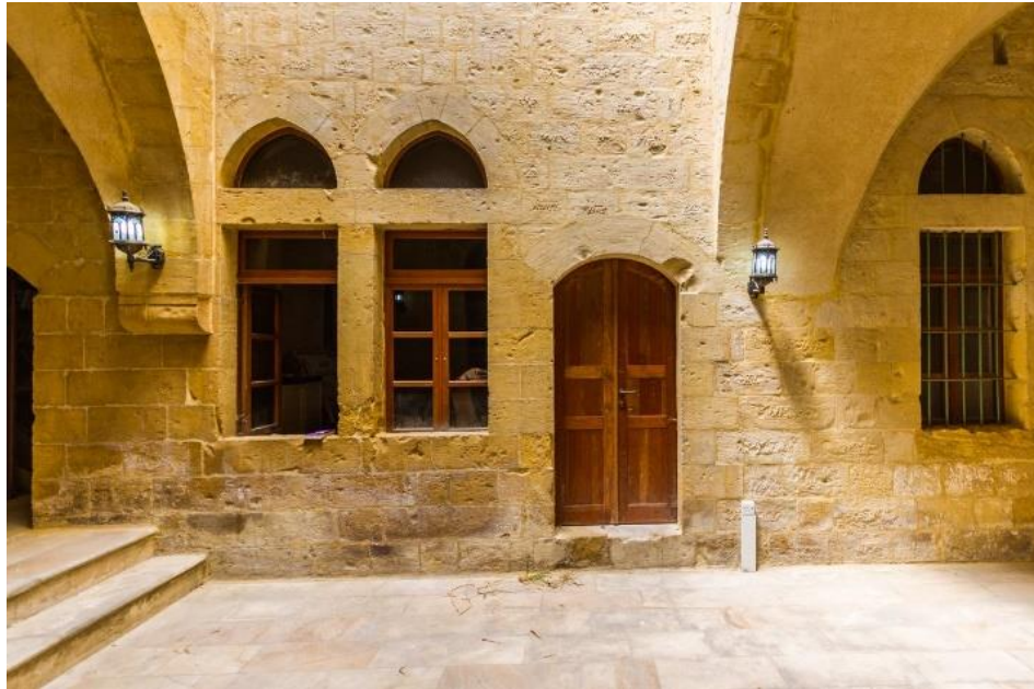
Figure 5.10 Example of a vernacular courthouse. Multiple tall-arched and narrow windows; and interior courtyards in vernacular houses provide excellent natural ventilation and cooling while also providing enhanced privacy for the family. (By Author)
