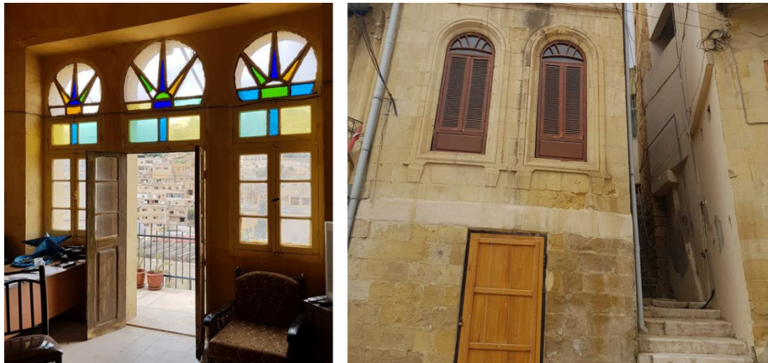
Figure 5.4 Examples of vernacular buildings in Salt city. Vernacular dwellings has their biggest windows positioned toward the street away from direct contact with neighbour's windows and courtyards (By Author)
