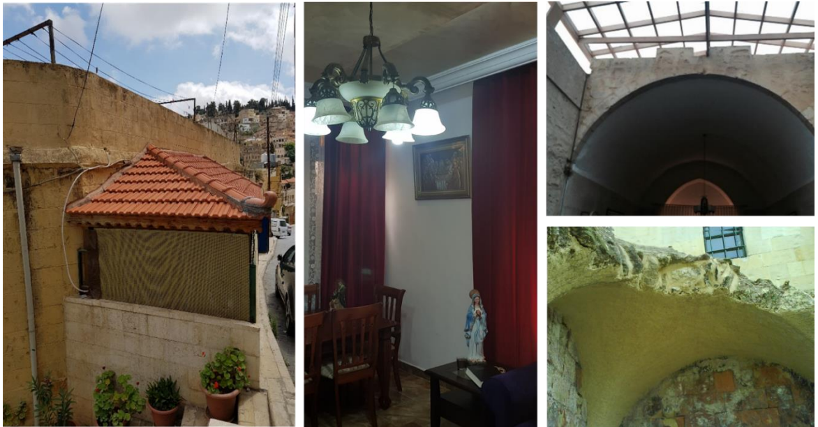
Figure 5.9 Examples of modifications to dwellings in Salt city. Changes were more common in Salt old dwellings as residents were trying to implement changes to make these old dwellings adapt to modern daily life. The most common changes include covering the central courtyard (top right), removing the masonry vaults and arcs, and replacing it with concrete slabs to add a second floor (bottom right). Changing the interior décor was also very common (centre). Less frequently were changes made to increase privacy (left).
