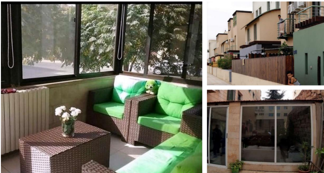
Figure 5.8 Examples of modifications to dwellings in King Abdulla city. In the modern development of Zarqa City, changes were more related to enhancing privacy, such as increasing the heights of the boundary walls (top right) and enclosing parts of the balcony and terrace (bottom right and left) with glass panels.
