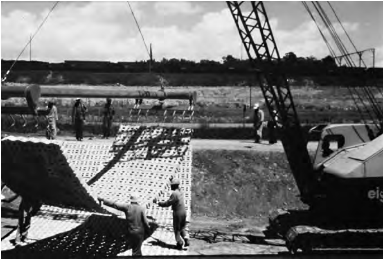
Photo 3: Flexible concrete grids provide a stable channel in densely built-up areas
