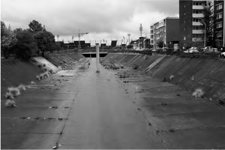
Photo 1: Concrete stabilisation of a channel
