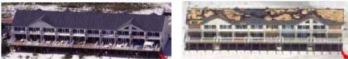
Figure 5.1 – Removal of panels of house in Florida, Hurricane Jeanne [USGS, 2005]
