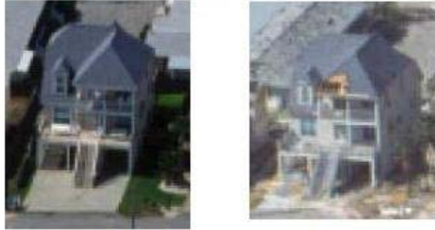
Figure 5.1 – Removal of panels of house in Florida, Hurricane Jeanne [USGS, 2005]
