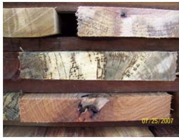
B. Extensive Degradation caused by Seawall
