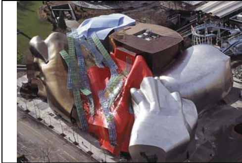
Figure 5.7 Exterior façade of the EMP project
