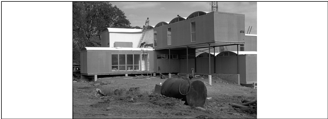
Figure 3.29 Oriental Masonic Gardens housing project in New Haven, CT 1968
