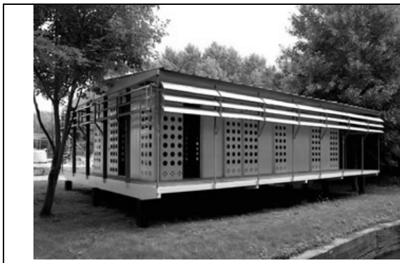
Figure 3.18 Exterior view of the Tropical House
