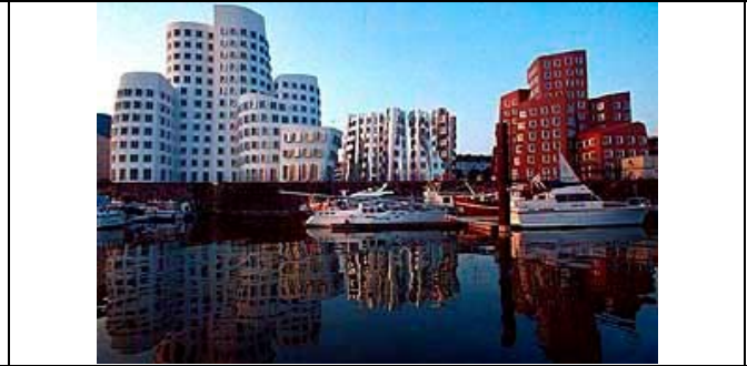
Figure 5.8 Façade of the Zollhof Towers in Germany
