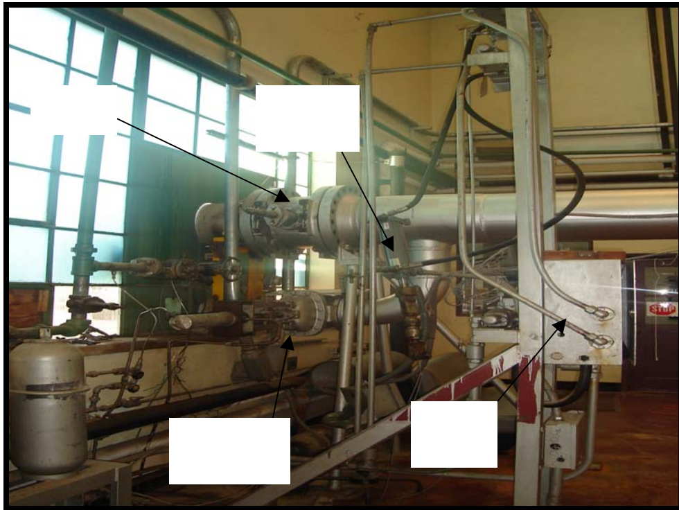
Figure 2.5 Butterfly Valve Control Mechanisms.
